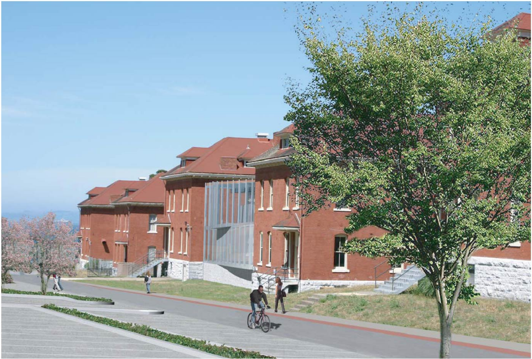
FIGURE 3: VIEW OF BUILDING 122 FROM TAYLOR STREET
