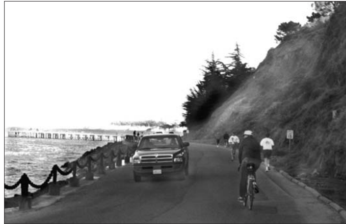
Figure 4-15. Existing Conditions at Golden Gate Promenade at Fort Point Extension
