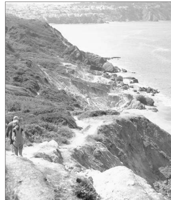
Figure C-11. Typical Location: Eroding and Hazardous Trail Edges
