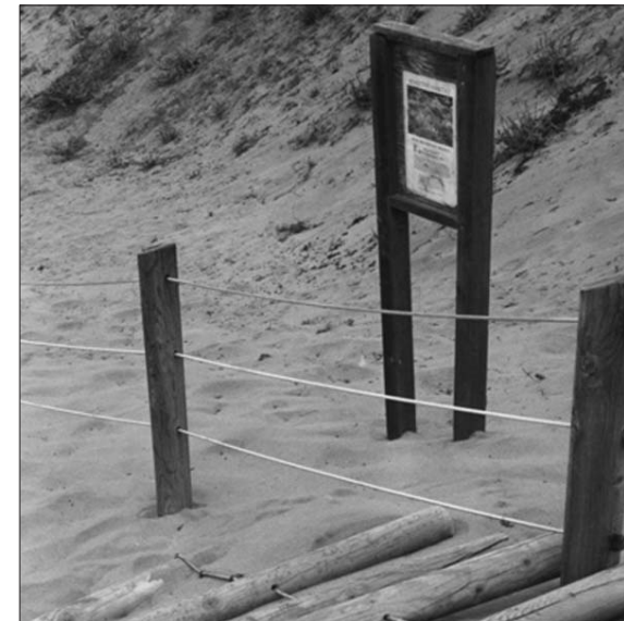
Figure C-16. Sand Ladder (BMP 6-2)
