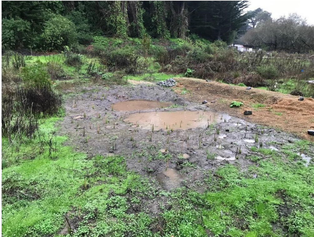
Image 8: north arm bioswale/retention basin, looking south east
