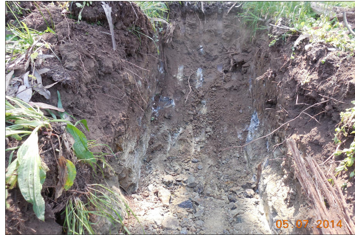
View of Trench. Note Scrape Marks from Backhoe Teeth on Bedrock.
