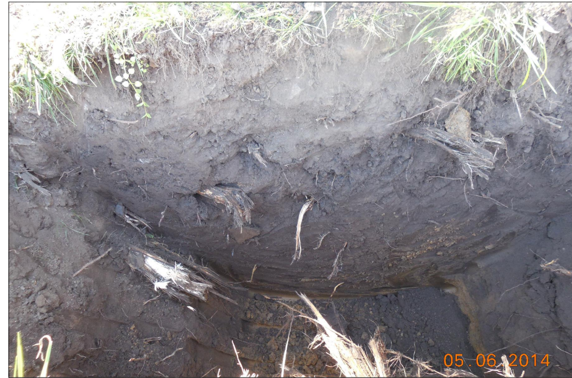
View of Trench with Tree Roots. Roots Subsequently Trimmed to Trench Edge with Approval of Trust.
