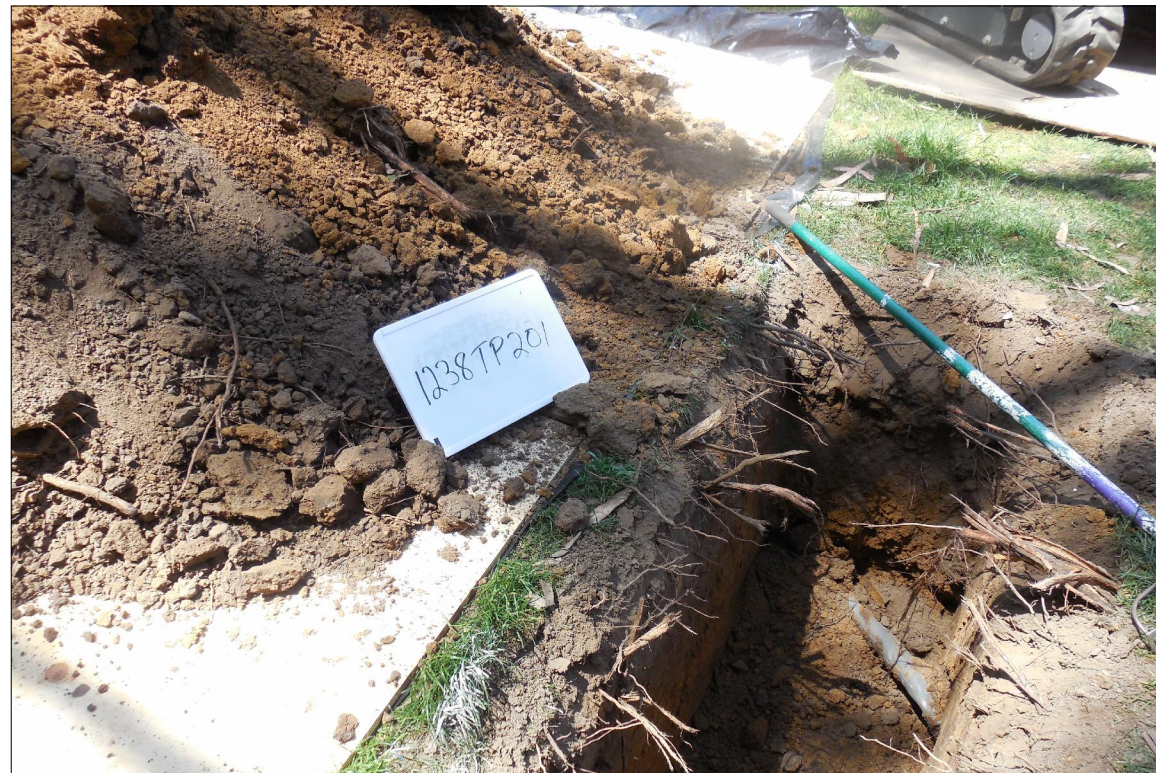
Spoils Pile, with Water Line Visible at North End of Trench. Rake on Surface Shows Trend of Pipe.
