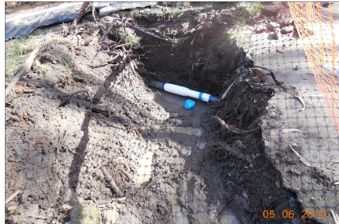
Trench with Repaired Water Pipe
