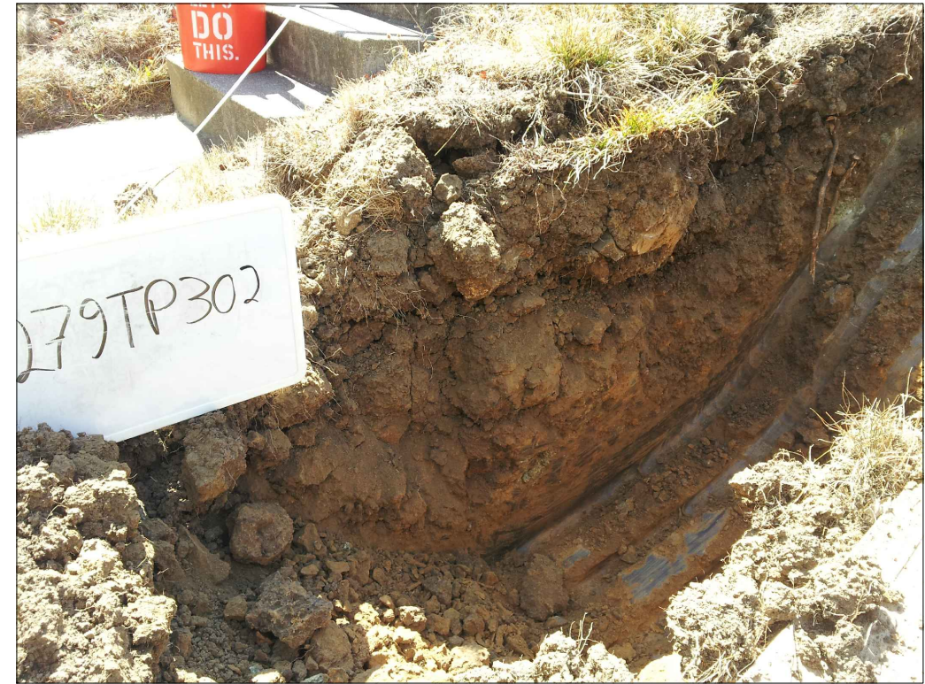
Excavating trench on slope.
