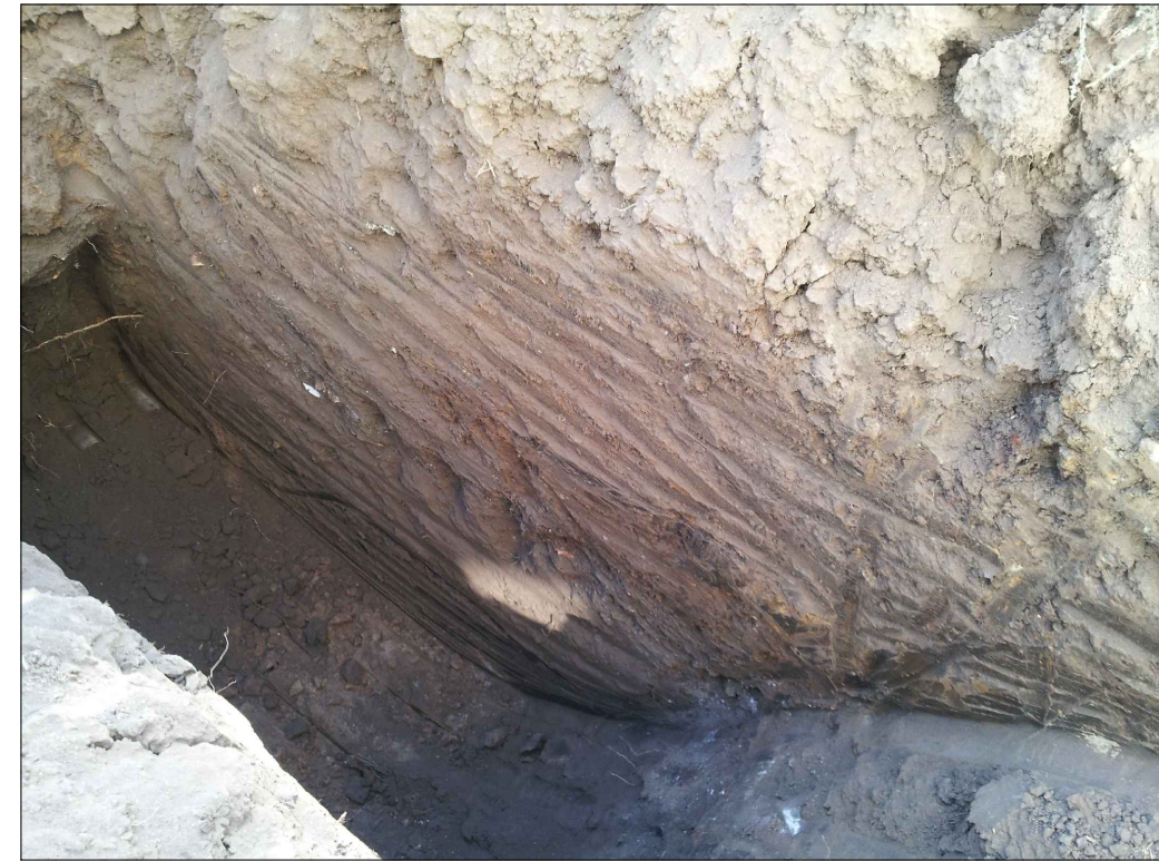
View inside trench. Note debris layer approximately 3 feet down.
