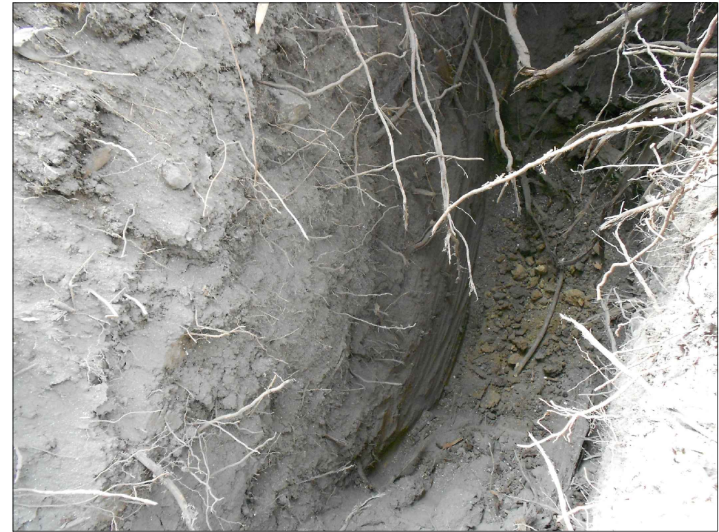
View inside trench. Note debris layer extends to native at bottom of trench.
