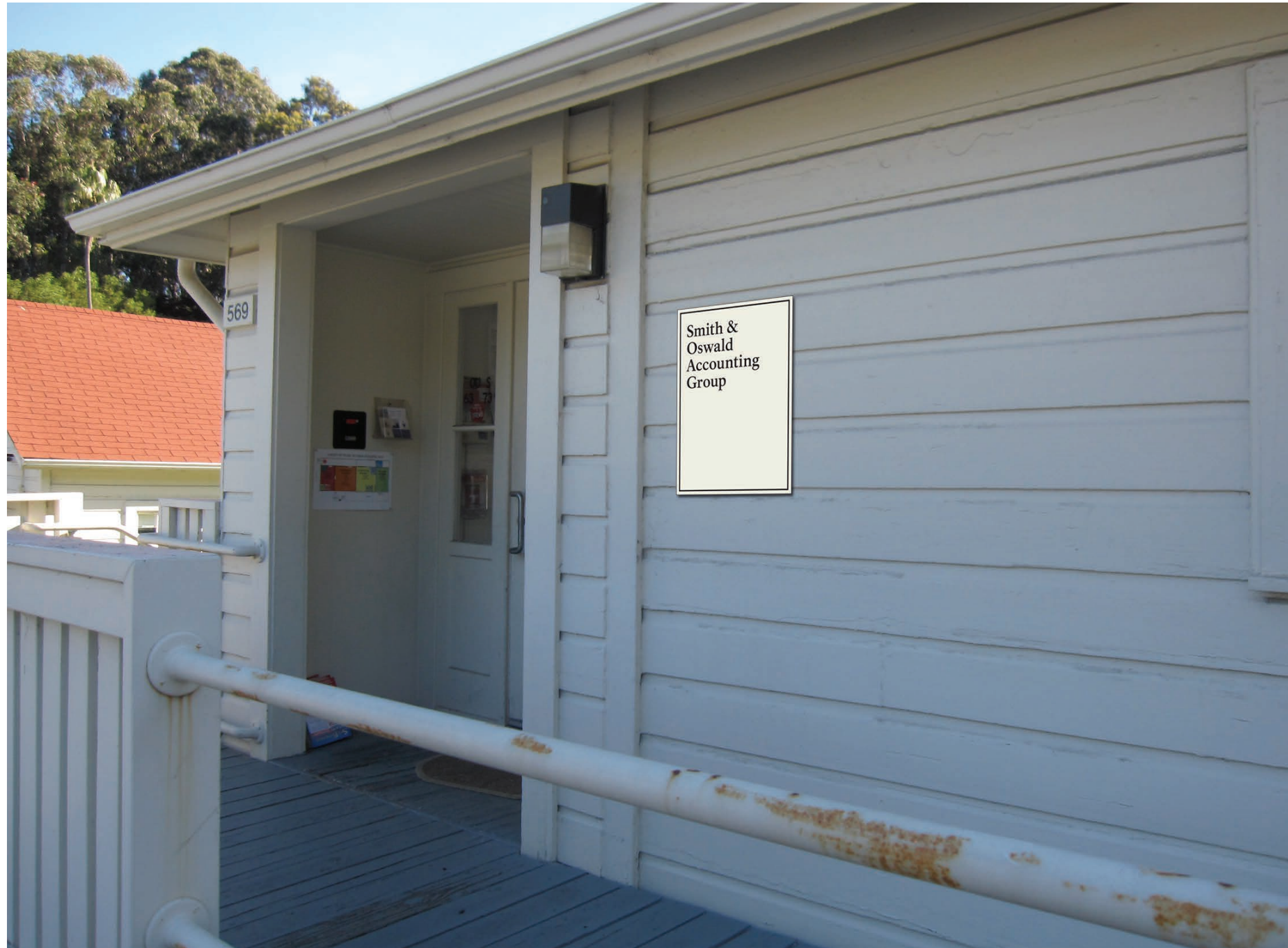
1 Sign Type WALL-MOUNTED TENANT ID : Office Tenant ID Sign Scale: Not to Scale
