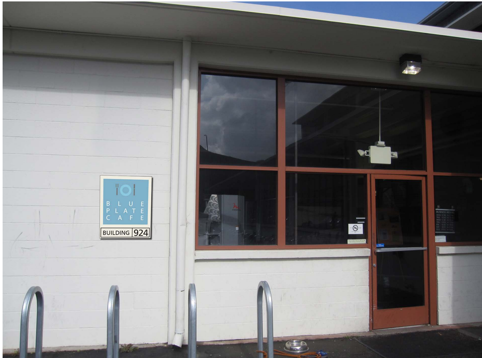
1 Sign Type CRISSY FIELD WALL-MOUNTED TENANT ID : Tenant Logo ID Scale: Not to Scale
