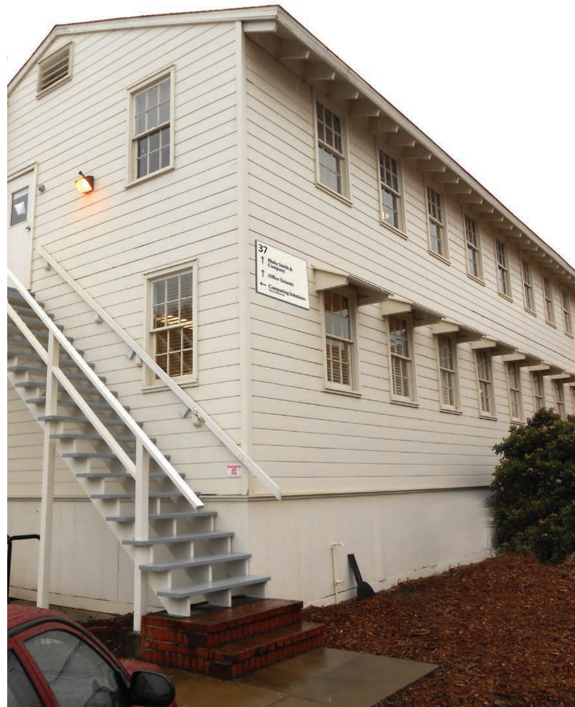
1 Sign Type WALL-MOUNTED TENANT ID: Tenant Directional Large Scale: Not to Scale
