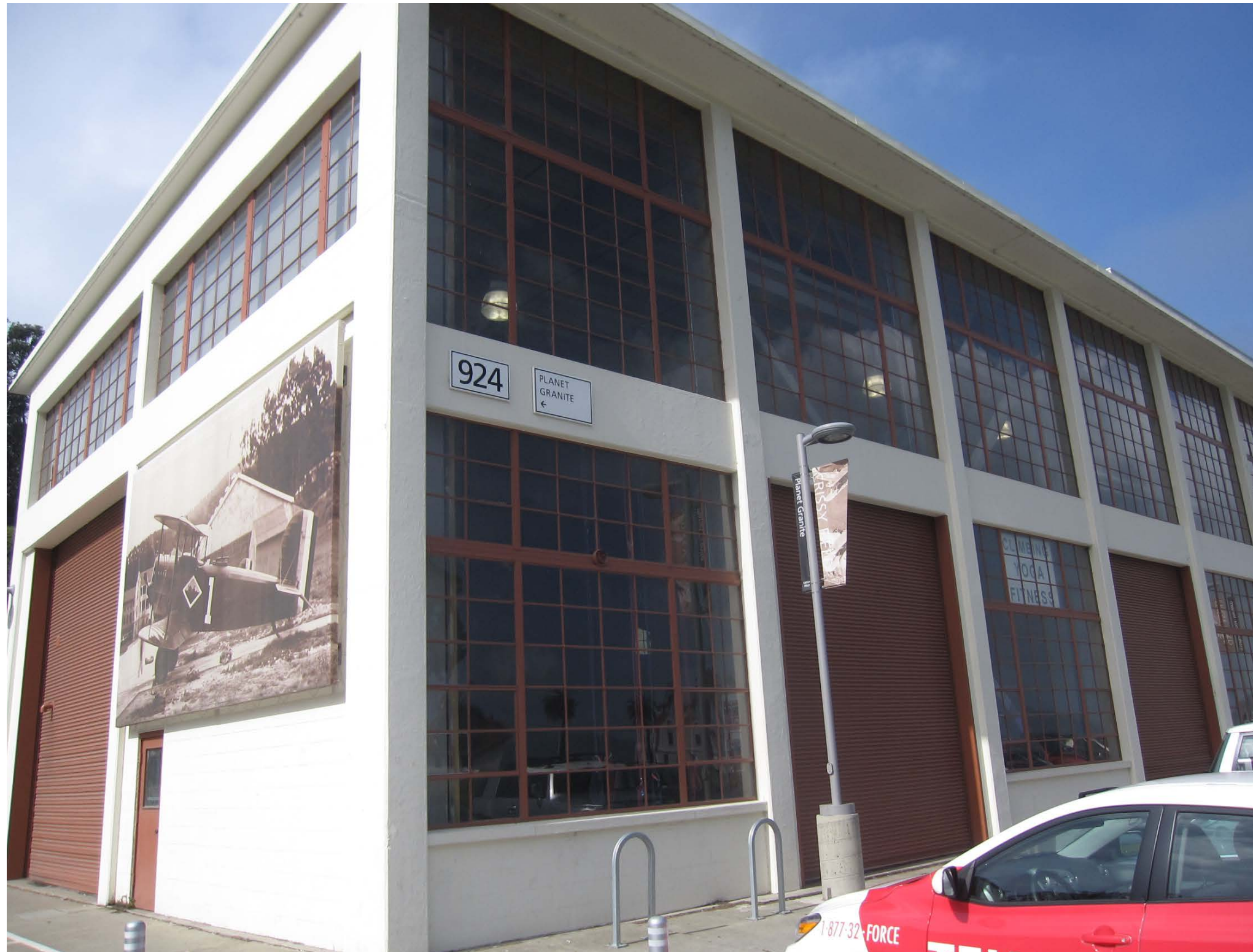
1 SignType CRISSY FIELD WALL-MOUNTED DIRECTIONAL: Tenant Directional Small Scale: Not to Scale
